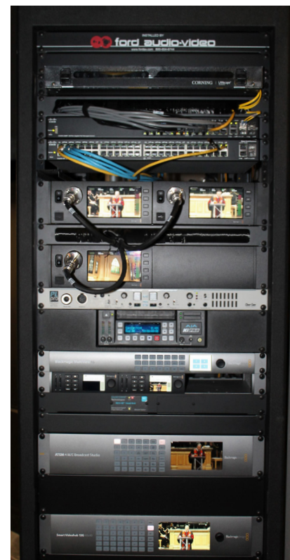
Equipment installed in the video room space at Asbury United Methodist Church in Tulsa, Oklahoma is shown in a rack, including a Blackmagic Design ATEM 4 M/E Broadcast Studio 4K production switcher.
